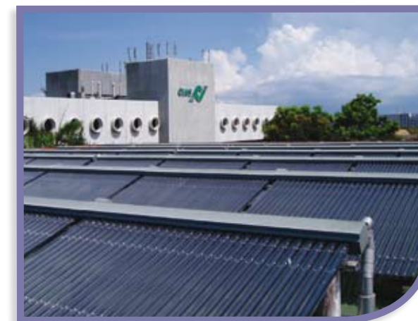
Changi Airport, Singapore. Largest solar thermal installation in South East Asia with more than 10,000 tubes.
