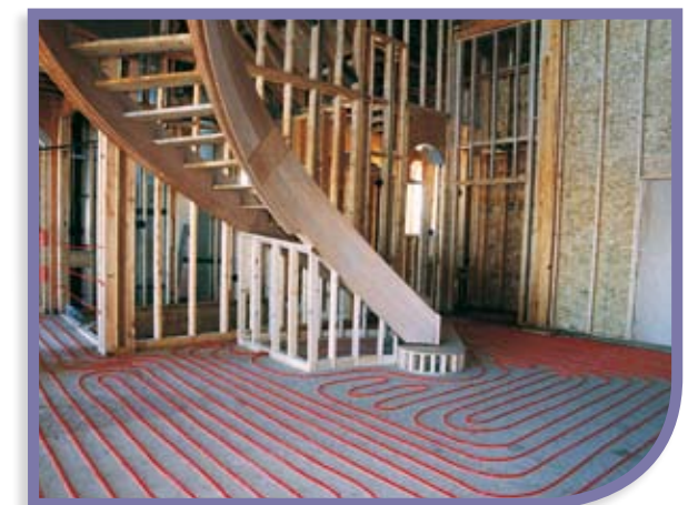
Radiant floor heating using a gyp-crete application.
